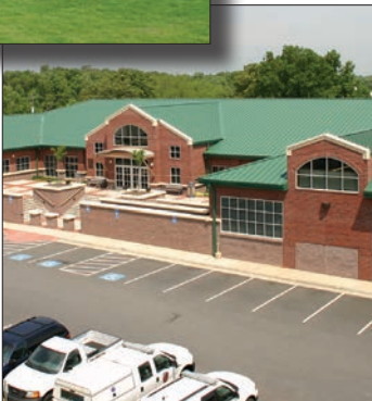
Public Safety Complex
